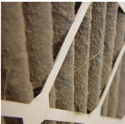
**A dirty filter, such as the one pictured above, can lead to a considerable loss in energy efficiency or much worse.**
