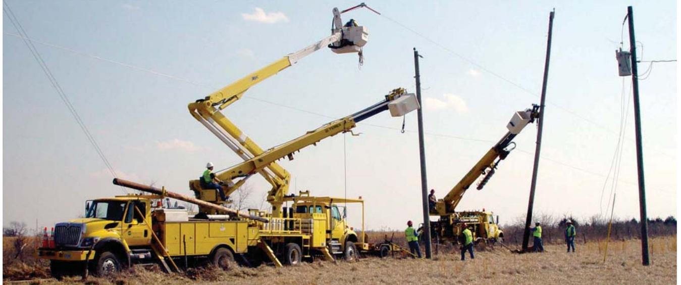
New-Mac Electric crews have already been plenty industrious in 2010. Thus far, New-Mac has accomplished three-phase conversion work on four of its substations, including Spring City (shown above), Spurgeon, Walkerville and Saratoga. Also underway, right-of-way clearing is occurring on the Neosho and Spurgeon substations.
